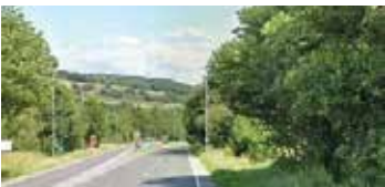
Accidents shut the bypass
